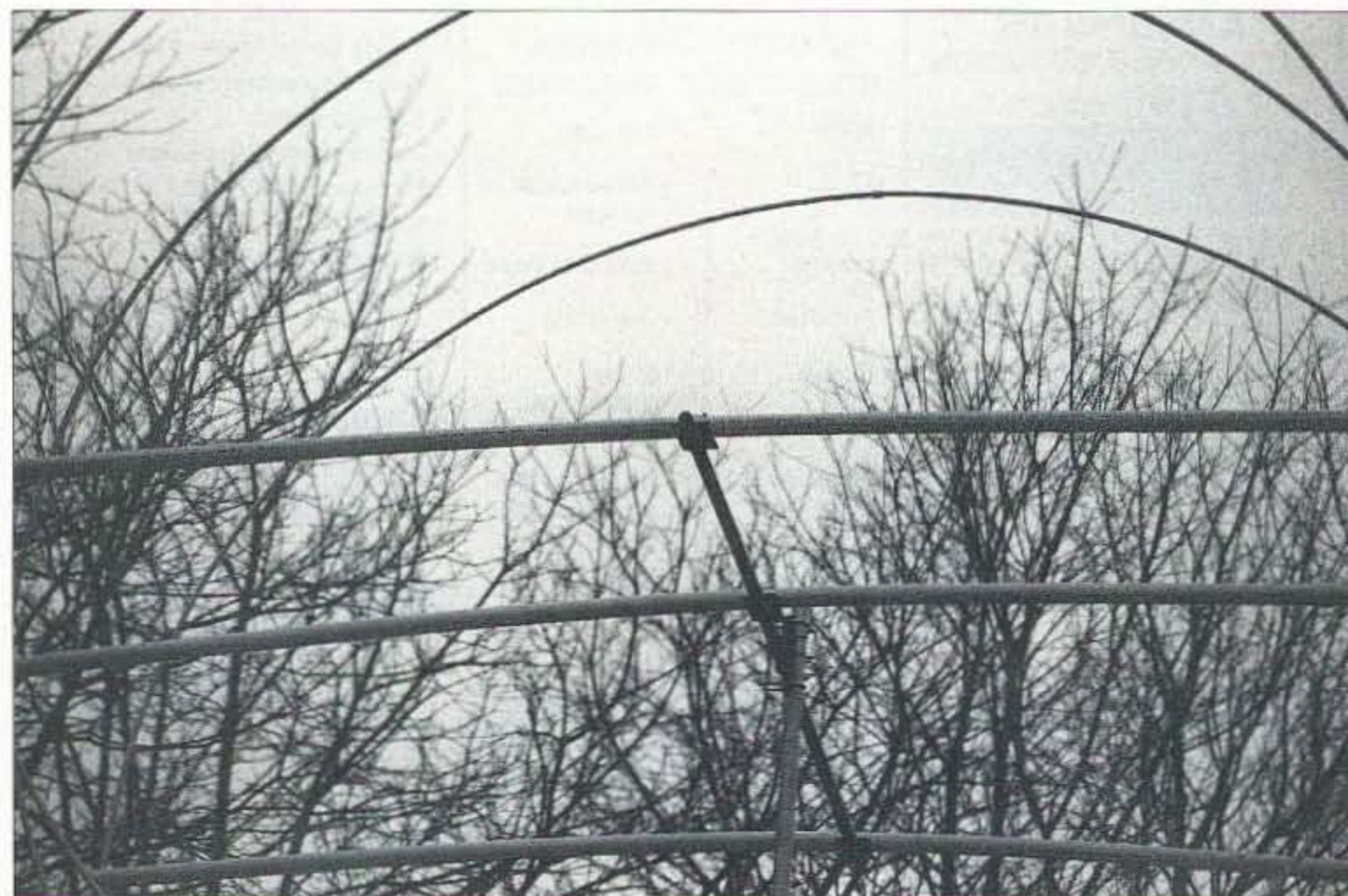
Photo B. Closer view of beam and elements.
